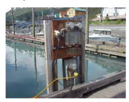
Most of the supply side of the electrical distribution system on shore has been upgraded and/or replaced to accommodate future upgrades. It is in good condition and should require only minor modification when float and electrical distribution systems are replaced or upgraded in the future.
