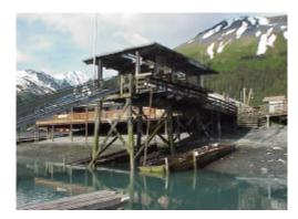
Most of the electrical system was originally installed using an upland trailer park system and worked for a short time. It was not a marine grade system and has gradually deteriorated to the point where it is unreliable and, in some areas, unsafe. Patches have been made over the years where feasible and in some cases service has been abandoned where economical repair could not be made. Customers have, with and without the harbor department's approval, installed electrical
